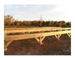
This shed foundation is good depending on the location and type of shed you build. It is also considered to be a post and beam foundation because the wood is not just sitting on the ground but it is attached to posts that are secured in the ground. The wood has to be pressure treated to withstand the moisture. Furthermore, posts are to be secured properly at the right depth for the weight of your structure so you do not have a leaning shed.
