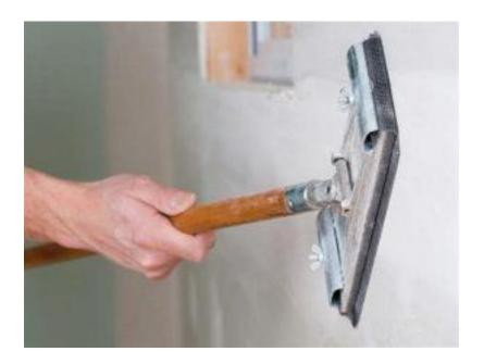
Once the compound is dry and uniformly white, then it is time to sand the drywall. Using a pole sander and a medium grit abrasive sand only the compound areas to where they are smooth. Don't sand it too much or you will sand down to the seam tape and you will have to do the process all over.
