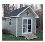
Cement siding is made from cement, sand and cellulose fibers and is a very durable siding. It installs similar to the wood siding and has the advantages of being more durable and resistant to water, fire and insects. However, it is a little brittle so it can crack upon impact. Also, there are special tools to cutting the boards and the create a lot of dust when cutting. The most common name in cement siding is HardiePlank siding.
