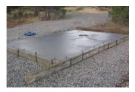
This is the strongest shed foundation construction and can withstand a full load contact. It is a great foundation for sheds with machinery. Therefore, if your shed is for equipment or a car then this is the one you want. With the concrete slab, you do have to be careful if the slab is much larger than your shed. If that is the case, then you run the risk of water resting on the slab and water damage to your shed. Think about your future water drainage. Read more in depth description below.
