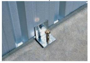
Brackets will be attached to the inside of the shed with expansion bolts or masonry screws. The bottom plate of the bracket is secured to the
