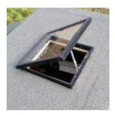
There are many different options with a venting skylight as some of the skylights can be automatic open or manual open. There is a solar powered skylight too. The automatic skylights will open and shut depending on the heat and the need for ventilation.
