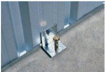
Brackets are easily secured to the shed by expansion bolts or screws. However, the brackets can be secured to the concrete foundation with either masonry screws or expansion bolts. If the bracket is an L Bracket on the inside, then I recommend expansion bolts. As noted above, drill the hole to the right size and depth for the expansion bolt. Place the bracket over the hole and then attach the expansion bolt. Next, attach the bracket to the shed with the proper
