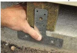
Side plates are kind of a retrofit and again are on the outside of the shed. For instance, the shed is built on a concrete foundation and the foundation is above ground level. This would allow one to attach a side plate to the foundation and the other end to the shed. You would use masonry screws for the concrete and galvanized screws for the shed attachment to the side plate. Galvanized screws will not rust so are better options on the outside.
