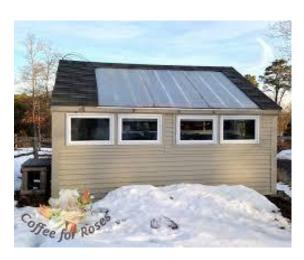
If you are using your shed for gardening or potting, then you may want to think about windows on the roof to allow sunlight into your shed. It will help with the plants for sure. You can use glass or Polycarbonate sheets. I recommend the Polycarbonate sheets because they are tougher than glass and can withstand the weather elements better. If you put the sheets on the wall and the roof then you can build your shed into it's own greenhouse.
