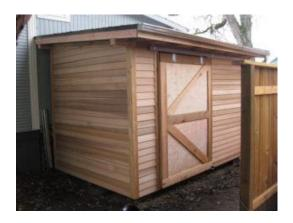
Dual Opening Shed Door Options: These doors open up together or one at a time. Very useful for sheds with lawn equipment or if you need a really large doorway to get any other equipment in or out of the shed.
